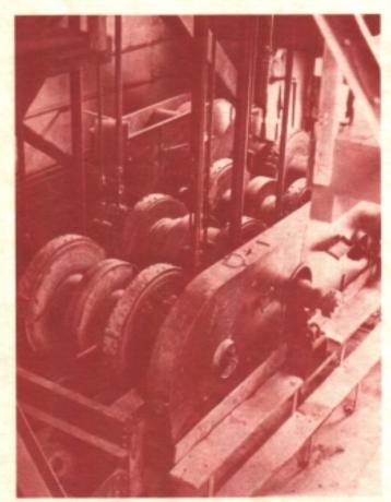
Winches and cables under the control room maneuvered the dredge on its 4.5 mile trek through the Goldstream Valley.
