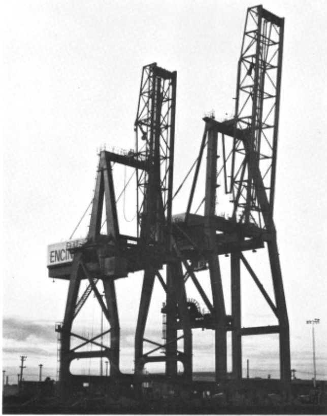
1959 and 1981 vintage PACECO container cranes as they appear today at Encinal Terminals.
