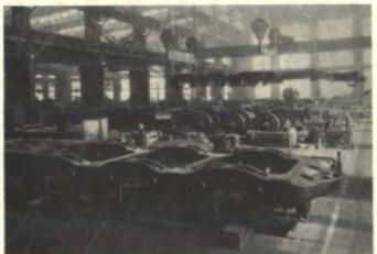
GG1 frames—note workers at left, center, and right for scale. Note 1-piece cast frame on overhead hooks — each GG1 has 2 frames, articulated by center hinge.
