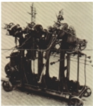
AN EARLY ATTEMPT AT AUTOMATING THE BULB-BLOWING PROCESS RESULTED IN THIS ODD-LOOKING MACHINE. THE AIR WAS STILL SUPPLIED BY LUNG POWER
