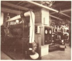
This heat pump, a part of the new installation, has the capacity to run 300 tons of refrigeration. It is one of two heat pumps which heat and  $_{\rm COOl}$  the Commonwealth Building. When both pumps are running, the system can handle 700 tons of refrigeration.
