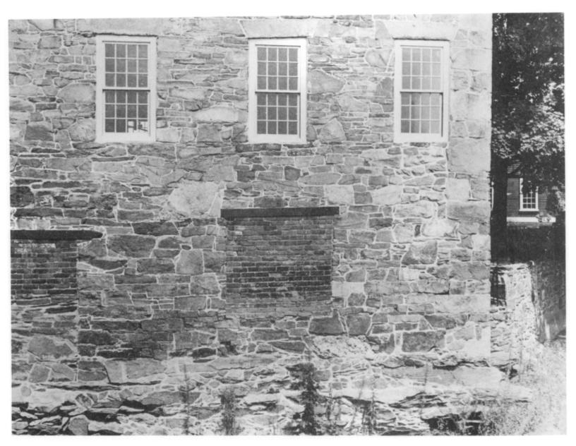
Cast Iron Shafting Used as Lintels
