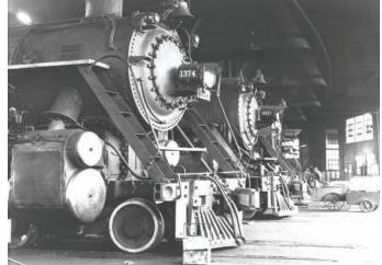
Steam locomotives in the Roundhouse. The smoke jacks are visible above the engines.
