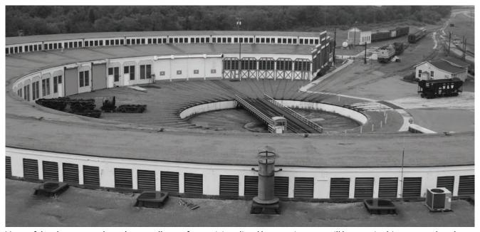
Many of the changes made to the roundhouse for servicing diesel locomotives can still be seen in this present-day photo, including the swinging wooden doors installed on stalls 33-37. The roll-up steel doors on stalls 29-32 were added in 1968.
