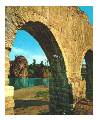
Noria al-Sihyuniyya: Together with the preceding one, at the same end of the dam, this is a single wheel noria of medium diameter of about 10 m (33 feet). It was rebuilt in 1981 and restored in 1988.
