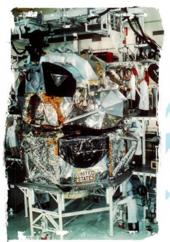
bartment, ascent engine, an electronic equipment bay, and a tank section. The descent to the lunar surface, the landing itself, and the eventual rendezvous with the Command Module are all controlled from the ascent stage.
