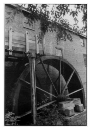
Around the outside of the wheel are sixty buckets inclined at an angle to catch water falling from the flume above. Each bucket holds approximately fifteen gallons (or 125 pounds) of water. The weight of water filling the buckets turns the waterwheel in a clockwise direction (when seen from outside the mill) and produces up to twenty-six horsepower. The waterwheel turning outside at a rate of 10 rpm spins the top grinding stones inside at 100 rpm.
