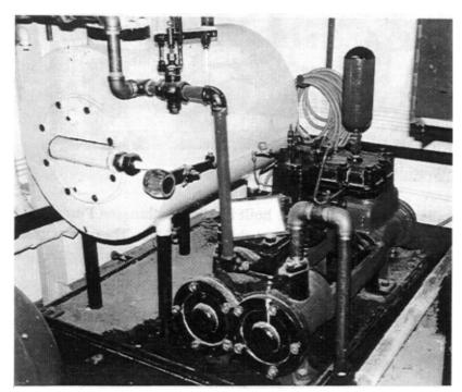
Engine #23 Gravity Return Pump
