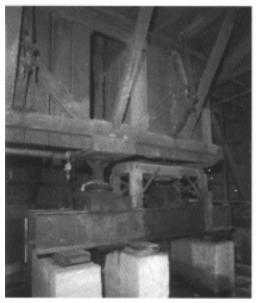
Ground floor view of the double box press which rotates on a center bearing post with hydraulic press block and cylinder under the box on the left. *Courtesy Richard Hofmeister, Smithsonian Institution*
