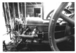
125 hp Bessemer Type IV oil engine installed in 1925. *Courtesy Doug Box, Doug Box Photography*
