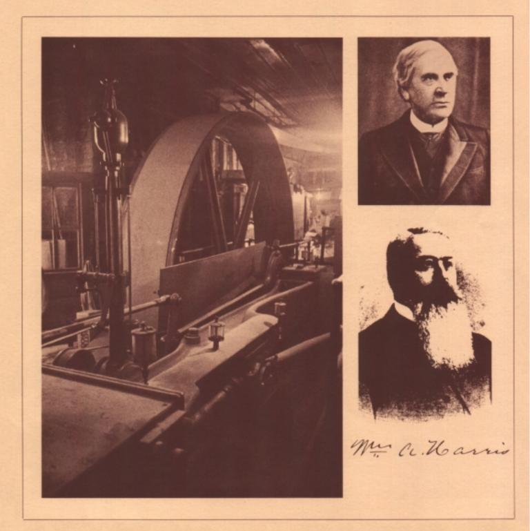
Sometime during 1977 the old 350 horsepower Harris-Corliss engine at the Randall Brothers Co. was retired from its job as a prime mover for the woodworking plant. Retirement did not come because of the age of the engine, over 80 years, but because of the U.S. Environmental Protection Agency's concern over the smoke from the boiler smokestacks. The engine was still, and is to this day, in perfect working order.
